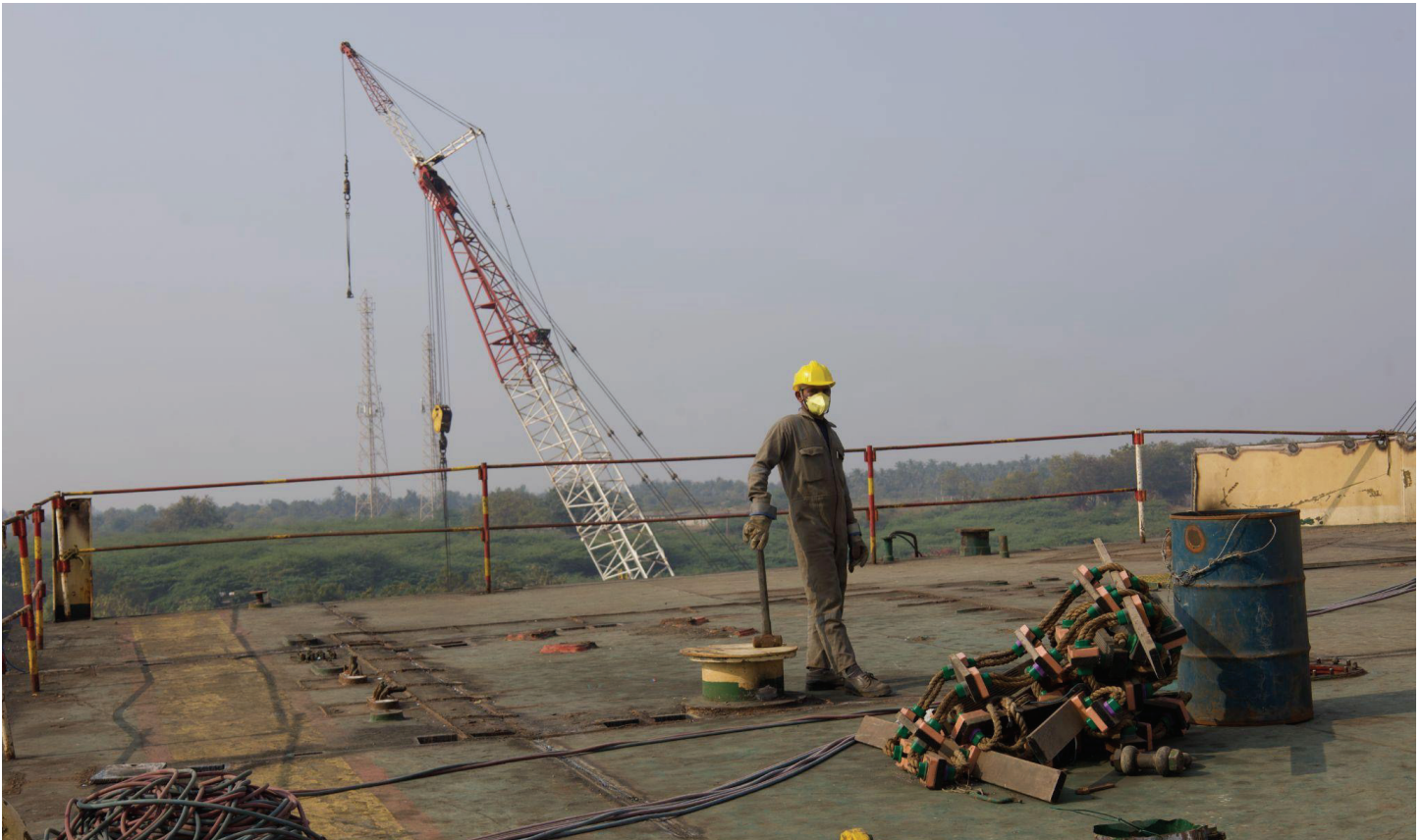
Figure 7. Worker on vessel during primary cutting Photo: Author fieldwork, Alang (Feb 2026).
