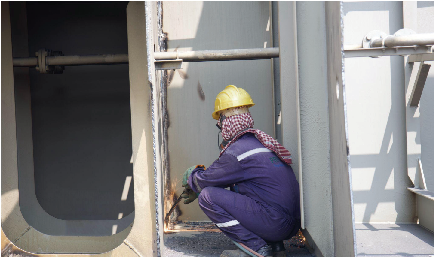
Figure 10. Secondary cutting operations on impermeable flooring. Photo: Author fieldwork, Alang (Feb 2026).
